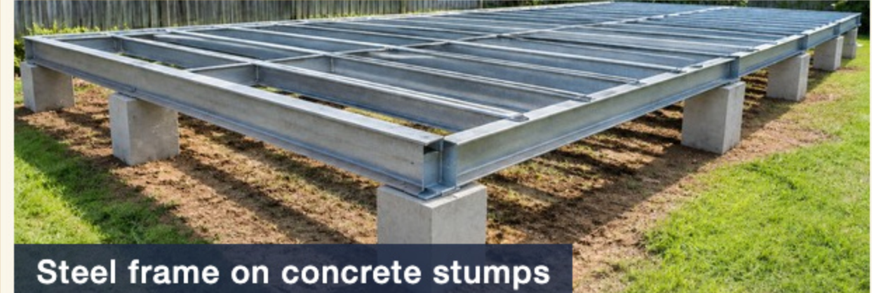
Steel frame on concrete stumps
